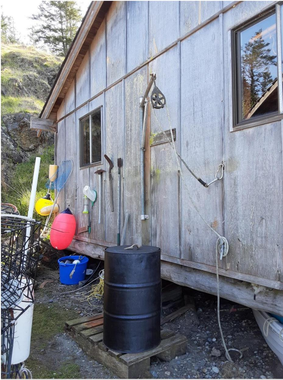
We have a new (re-furbished) salt-ease container to replace the damaged barrel. UV rays made it brittle and prone to breakage. In addition, we have installed a crane and pulley system. This should make it much easier to lift your skiff motors when doing your final rinse before departing.
